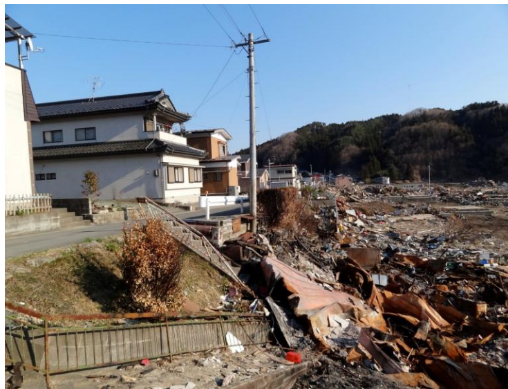
Photo 1 Contrast between the elevated district and lower districts of Tanohama
