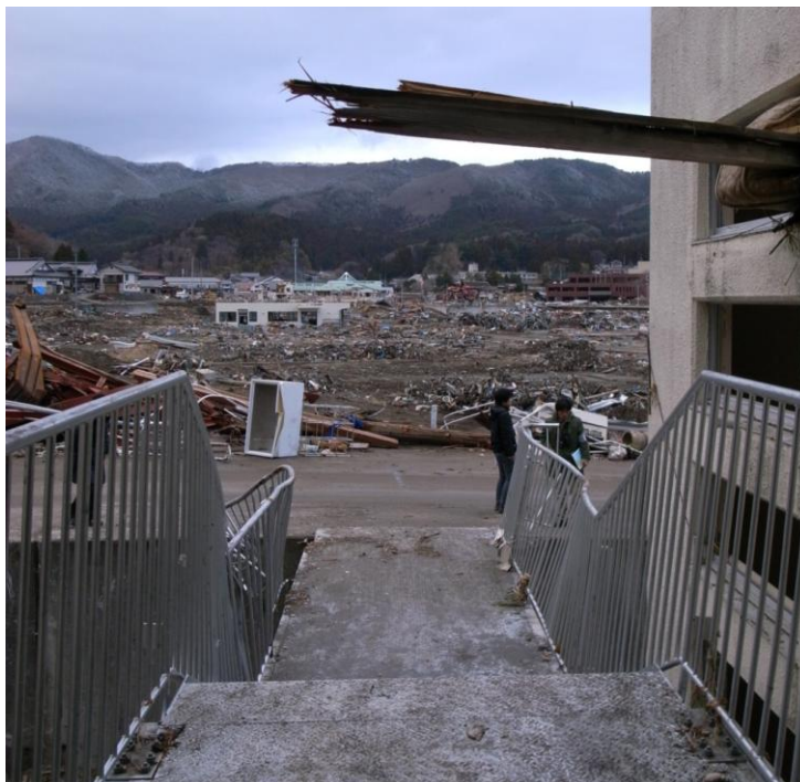
Photograph 2 Evacuation bridge at the Okirai Elementary School
