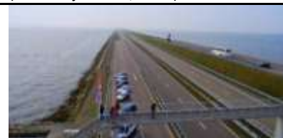
Enclosure of Zuyder Sea with a dam - Afsluitdijk at IJsselmeer (Author, 2012)
