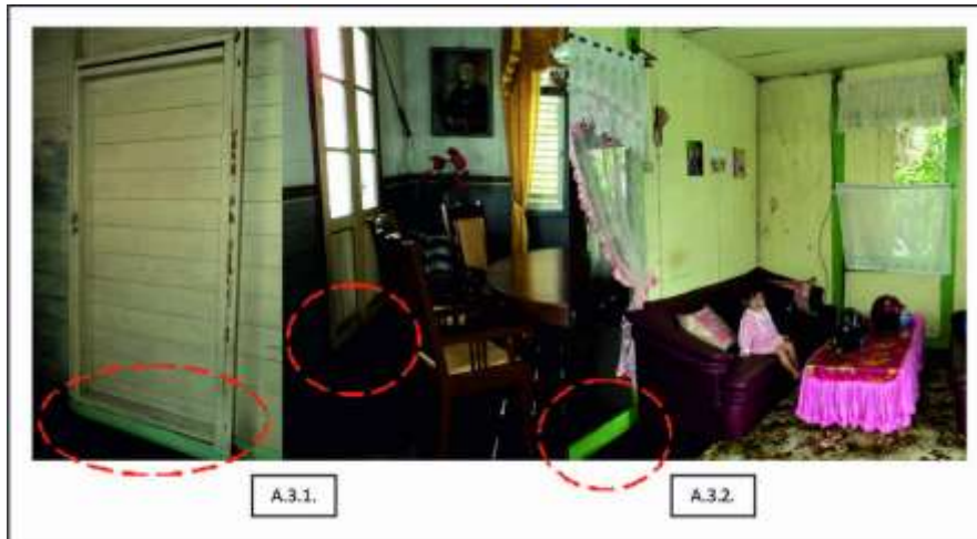
Figure 6. Beams above the floor as the boundaries of spaces found in the traditional Malay dwellings of West Kalimantan (photos were taken from the inside room of cases of A.3.1. and A.3.2.)
