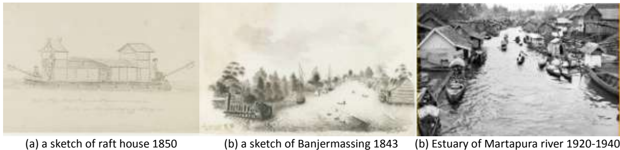
Source: (a-b) http://kitlv.pictura-dp.nl ; (c) www.tropenmuseum.nl Figure 7: Early river-based Settlements in Banjarmasin
