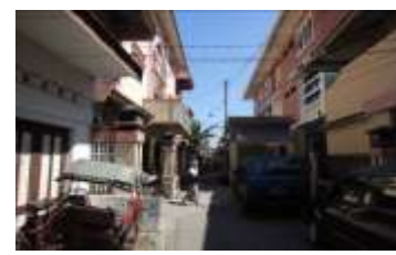
Modern storey Muallimat Madrasah in Islamic architecture among the narrow kampong roads
