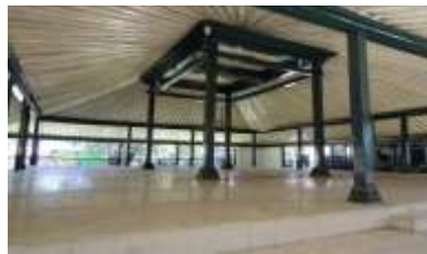
Main pillars and tumpang sari in the hall of Dhalem Notoprajan which are preserved as heritage architecture
