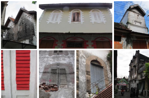
Figure 11. Grille and faux windows on the second floor of the building as well as aesthetic ornament as a tool of social status
