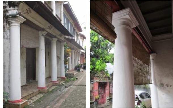
Figure 8. The application of Doric columns at the front halls of the buildings
