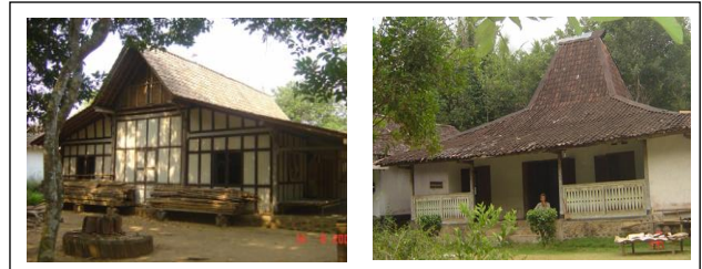
Figure 7 Traditional houses (Photo source: D.H. Rahmi, 2011)
