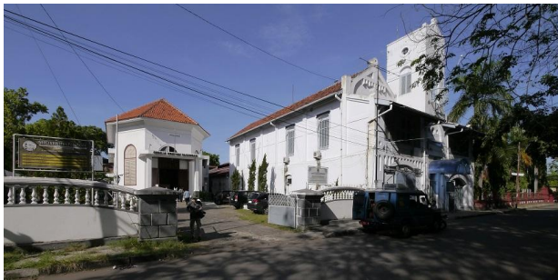
Figure 2. Gereja Kristen Pasundan, Cirebon, constructed in 1778 Source: field survey, 2014
