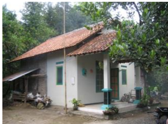
Figure 9. A core house in Kasongan after expansion (middle). The original core house is in front, painted a light color. The addition extends to the back, and is unfinished brick.
